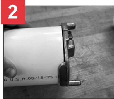
Chamfer (bevel) the end of the pipe 10° - 15°.
