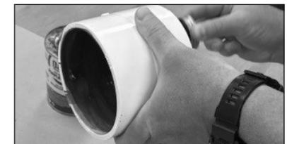
6. Working as quickly as possible, slide the repair coupling to the mark on the pipe that used the full length of the coupling to measure. Then, slide the repair coupling back down over both ends of pipe to the mark where you used half of the repair coupling to measure. A bead of cement will be present around the entire diameter of the pipe and coupling.
