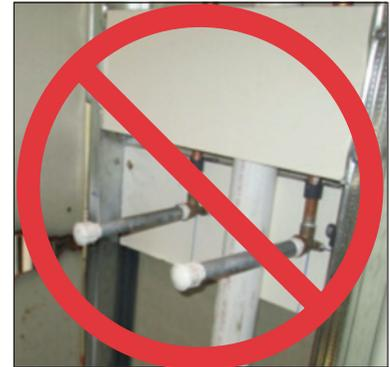
There are several problems with this application. First, the International and Uniform Plumbing Codes do not permit the use of PVC 40 pipe and fittings to be used in domestic water
