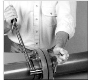
6. Use a torque wrench to tighten the bolts to the torque values shown below.
