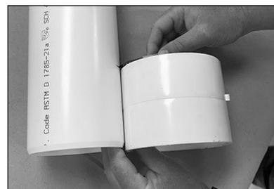
4. Apply primer to the inside of the repair coupling and between the marks and pipe ends on both pieces of pipe.
