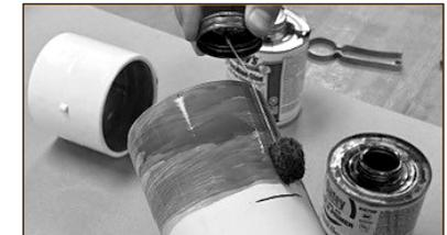
5. Apply solvent cement to the ID of the repair coupling and both ends of the pipe between the marks. Then, reapply cement to the ID of the repair coupling. Utilize heavy body cement for PVC and a medium body cement for ABS.
