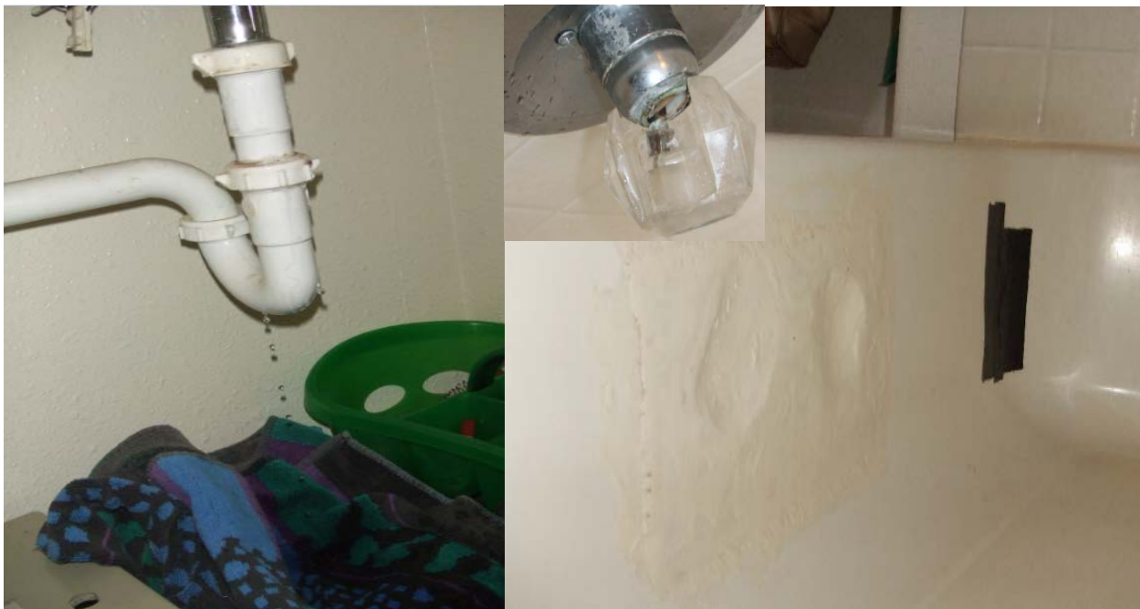
Photograph 8: One bathroom had a leaking sink pipe, a second bathroom had a broken shower faucet, and a third bathroom had a bathtub patched up with plaster and duct tape.
