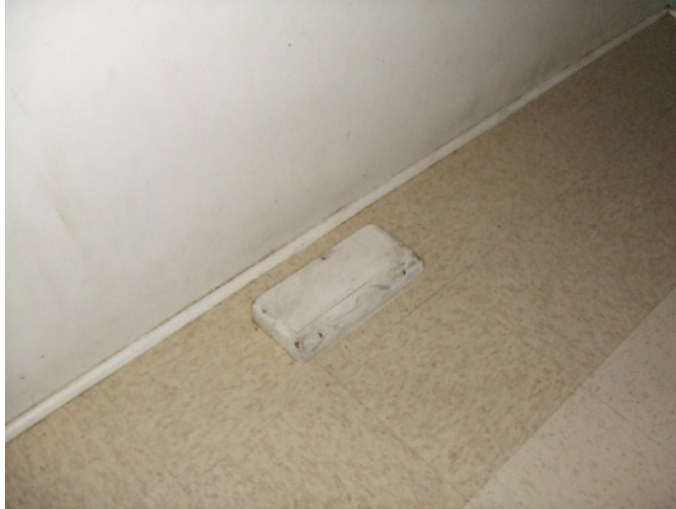
Photograph 11: An occupied bedroom's air vent was screwed shut, preventing air or heat from coming into the room, which did not ensure that the room temperature was being maintained at a reasonable level.
