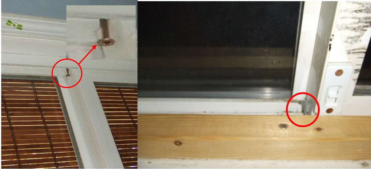
Photograph 17: Bedrooms' windows were screwed shut, preventing access in case of emergencies.
