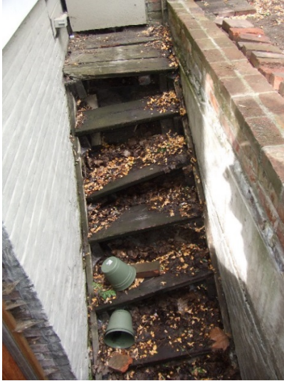
Photograph 7: A broken and decayed wood staircase leading to a basement was in disrepair and was accessible to children.
