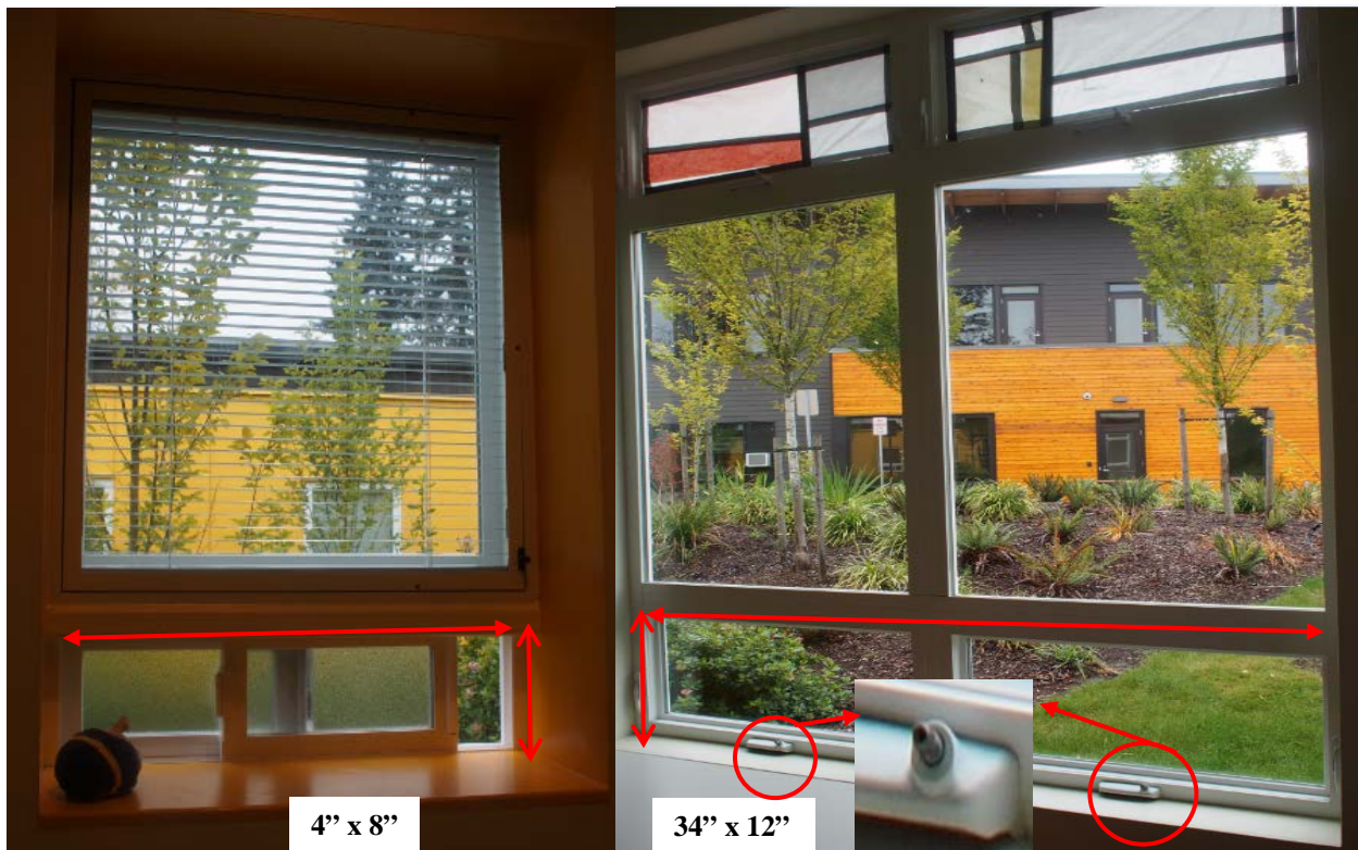
Photograph 16: The window openings in a bedroom (left) and living room (right) were too small to be accessed in case of emergencies, and the handles used to open the windows in the living room had been removed. The upper portions of the windows could not be opened.
