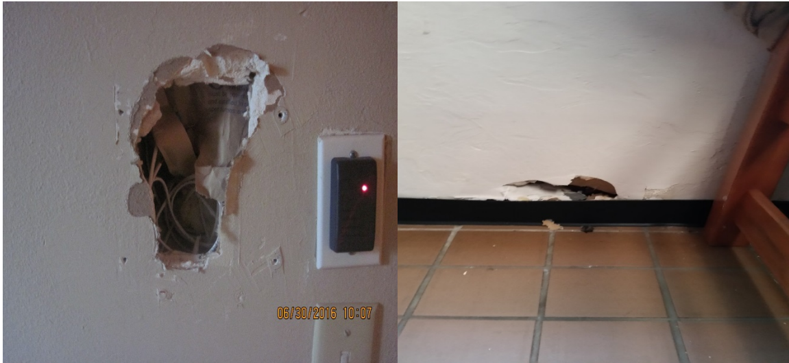
Photograph 7: Holes in facility walls, including one with exposed wiring.
