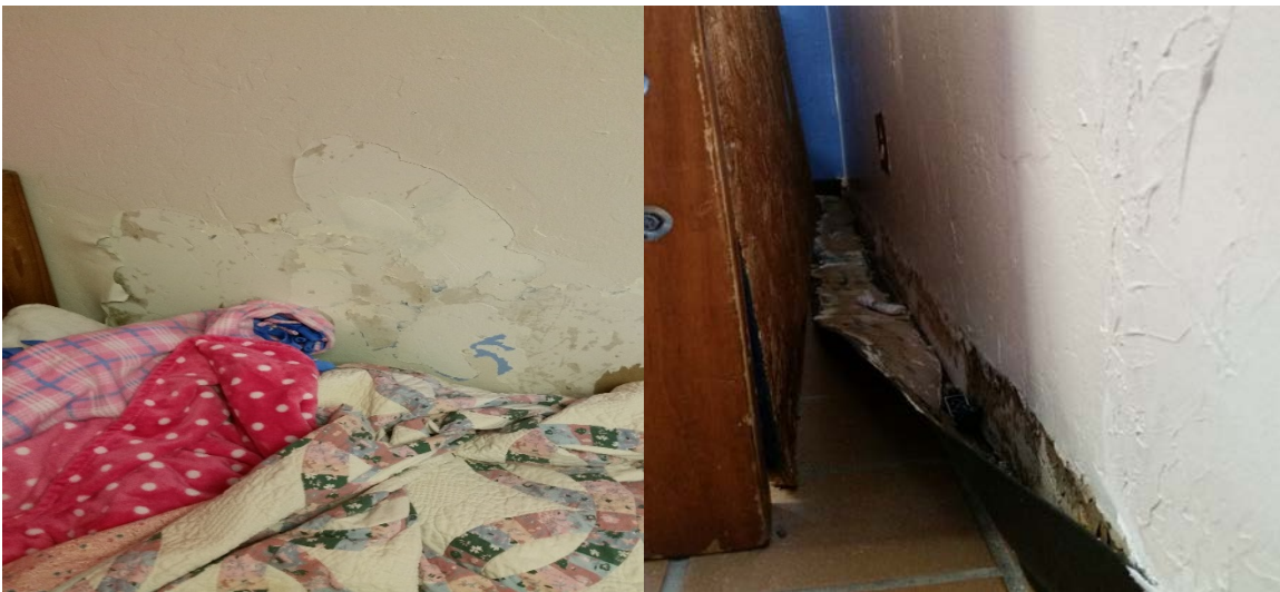
Photograph 6: Cracked or peeling paint found in various bedrooms at one facility.
