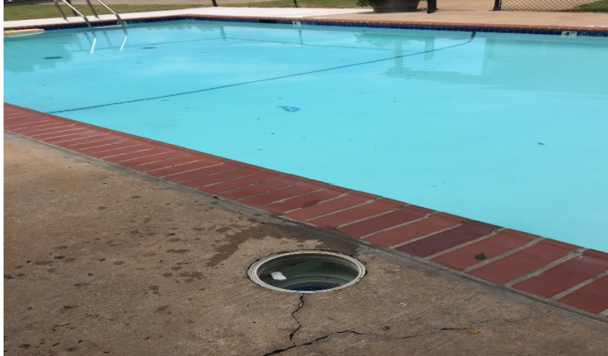
Photograph 9: One of the covers at a swimming pool (about 12 inches in diameter) was missing. During our walkthrough, five children were using the pool.
