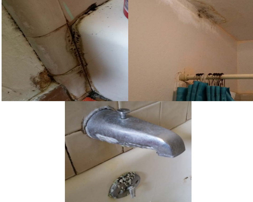
Photograph 15: Mold, mildew, and calcium buildup found in multiple bathrooms of one group home.
