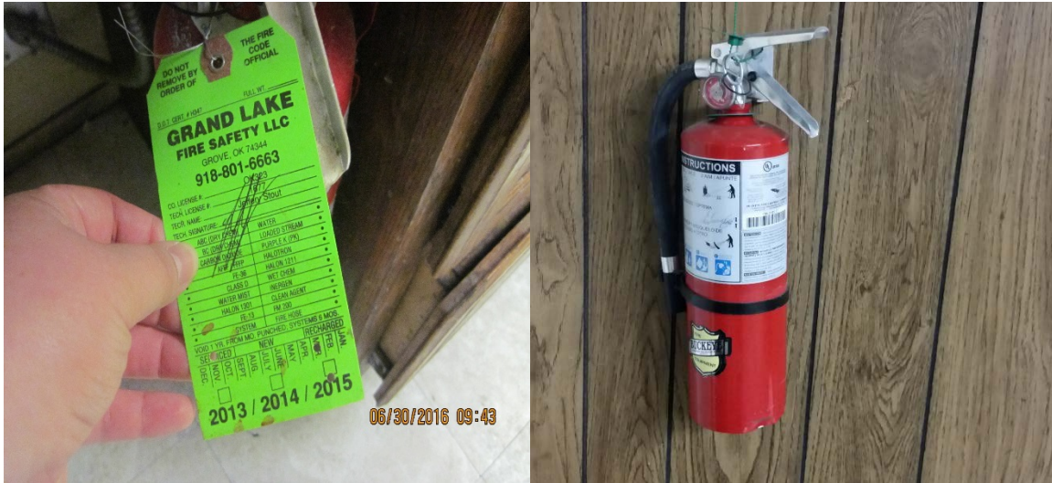
Photograph 11: An expired fire extinguisher and a fire extinguisher without a fire safety tag.
