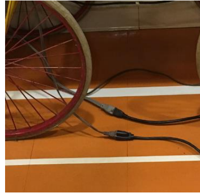
Photographs 6 and 7 (close-up): Extension cords were used as a substitute for fixed wiring.
