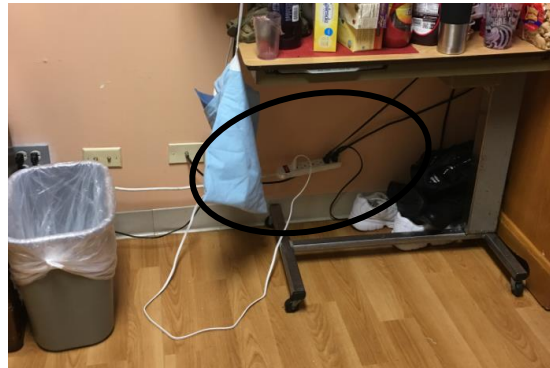
Photograph 8 (left): Power strip was unsafely connected to appliances near a water source. Photograph 9 (right): Power strip did not meet UL requirements and was used unsafely.
