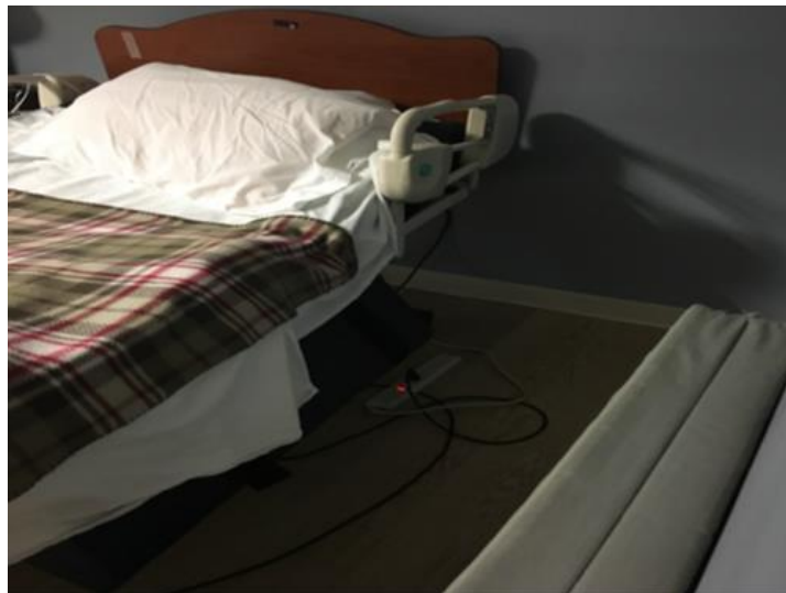
Photograph 10: Power strip did not meet UL requirements and was used on patient-care-related electrical equipment.
