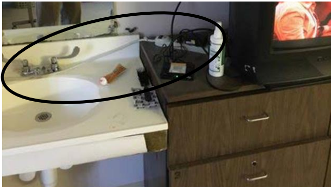
Photograph 8 (left): Power strip was unsafely connected to appliances near a water source. Photograph 9 (right): Power strip did not meet UL requirements and was used unsafely.
