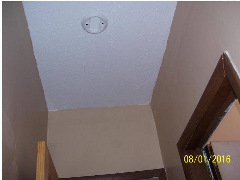
**Photograph 12: A smoke detector was missing.**
