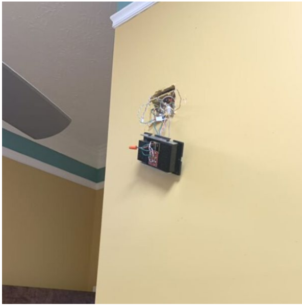
Photograph 5: Exposed Wiring.
