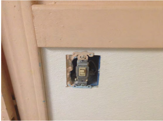
Photograph 13: Exposed electrical wiring.
