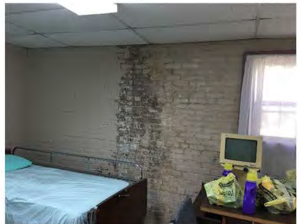
Photograph 2: Water damage and mold.
