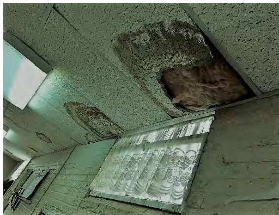
Photograph 8: Water damage and mold.
