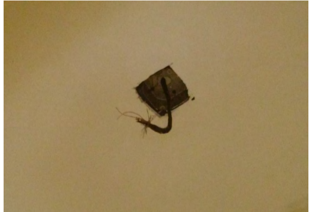
Photograph 14: Exposed electrical wiring.
