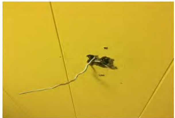
Photograph 4: Exposed electrical wiring.
