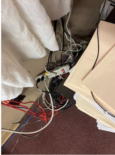
**Photograph 19:** Electrical wiring was “daisy chained.”
