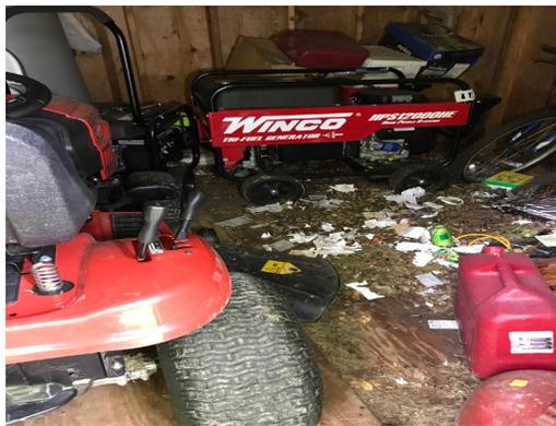
**Photograph 20:** A generator was stored in a wooden shed with full gas canisters. An animal was nesting in the shed.
