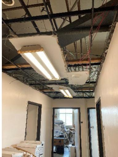
**Photograph 6 (left):** This emergency exit required a code for exit. **Photographs 7 and 8 (middle and right):** Ceiling tiles were missing or damaged.
