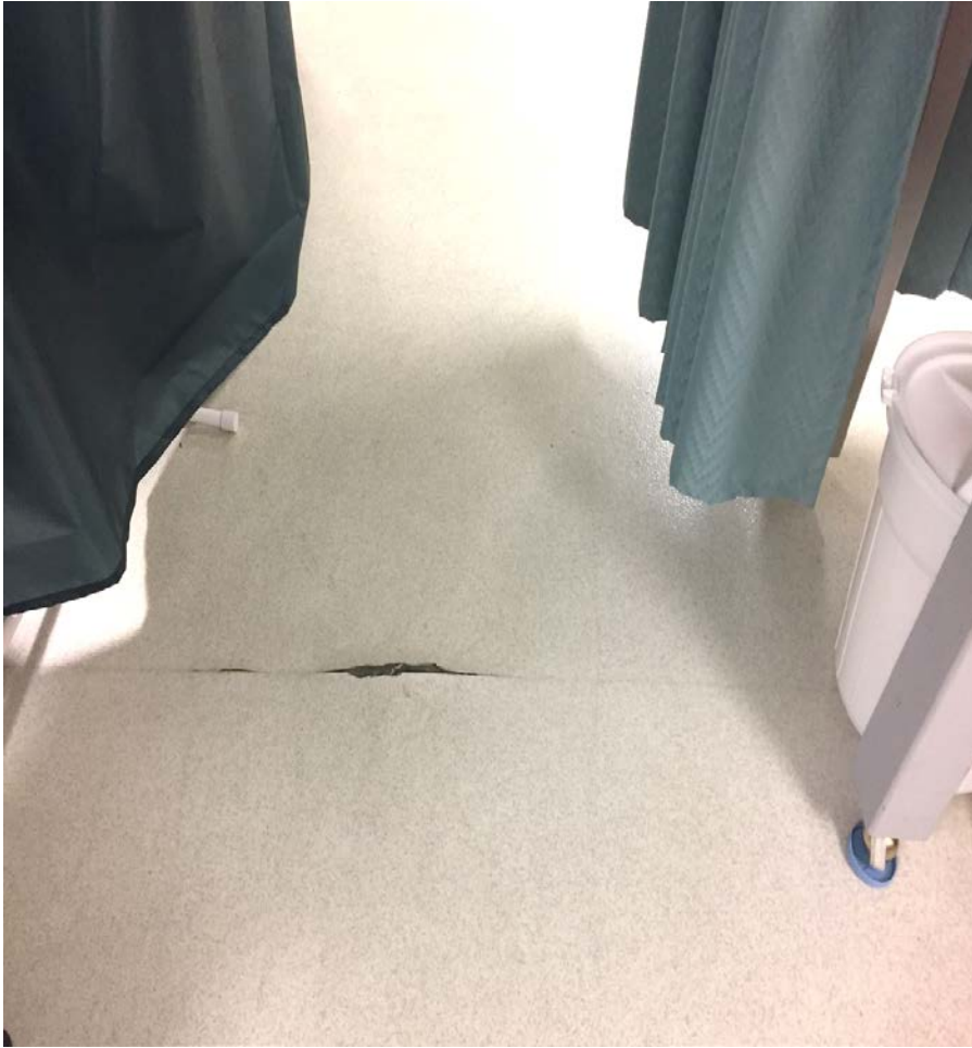
Photograph 1: Cracked linoleum flooring in triage room. Cracked flooring in medical treatment areas increases the risk that staff and patients could trip and fall resulting in injury and that the treatment area cannot be adequately cleaned and sanitized.
