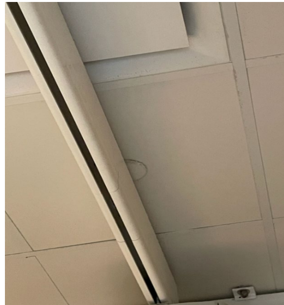
Blocked Sprinkler Head
