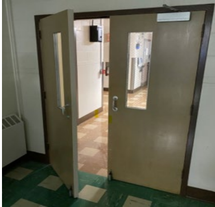
Photograph 3: Self-closing door stuck in an open position.
