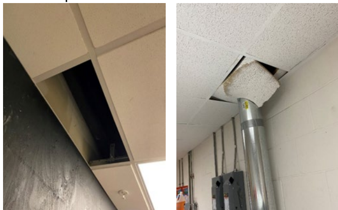
Photograph 1 (left): Missing ceiling tile. Photograph 2 (right): Broken ceiling tile.
