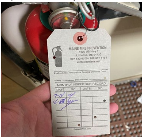
Photograph 4: Fire extinguisher month inspection tag identified during our unannounced site visit on November 19, 2024, was not filled out for September and October 2024.
