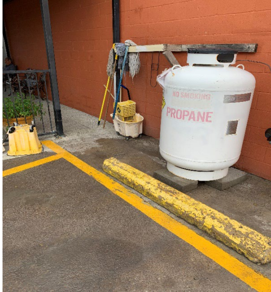
Photograph 3: Unsafe Conditions: Propane tank next to the smoking area.
